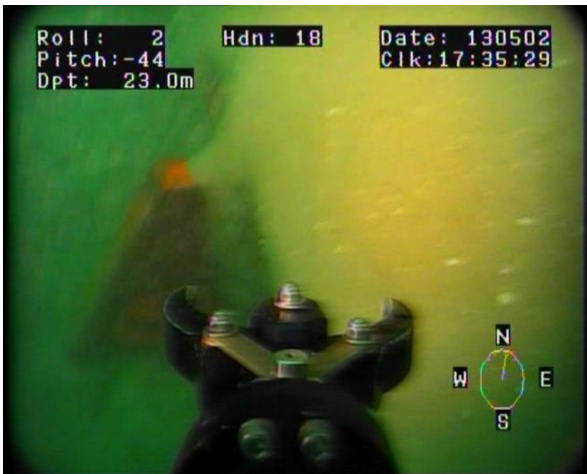
Figure F.5 VTG05_AC14_20130502_17h35m29s_Sand flowing over crown during pull.jpg
