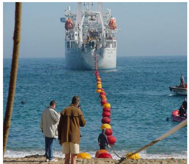
Landing the shore end of a submarine cable
